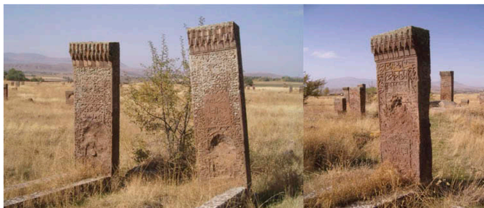
Figure 8. Eroded central sections of some stelae.
